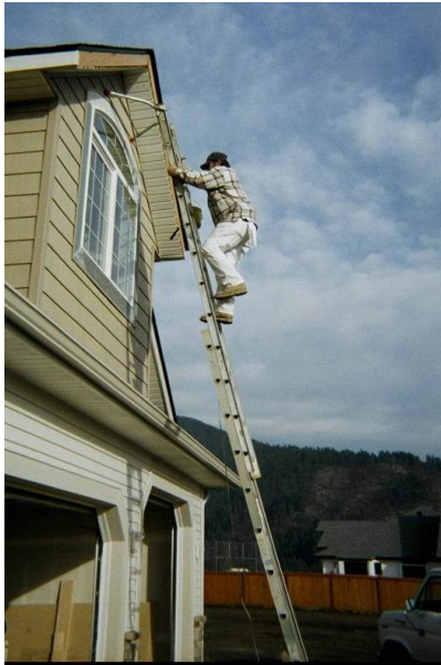
Works with 40 foot ladders
